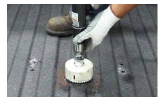
Step 4 - Use pilot hole to drill down, no measuring required
